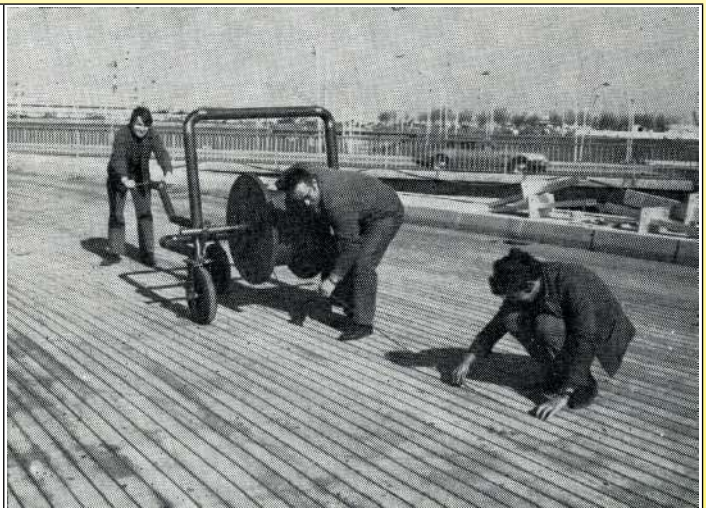
1968 Installation of the heating web on an access ramp to a bus parking platform, Orly airport near Paris ( Electric floor heating, by Robert Félix, 1971, Ultimheat Museum* )
